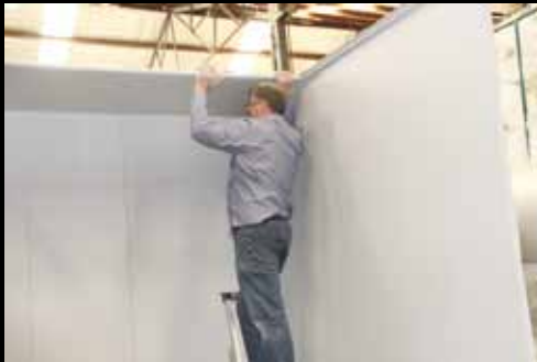
▲ Install walls and ceilings with the greatest of ease.
